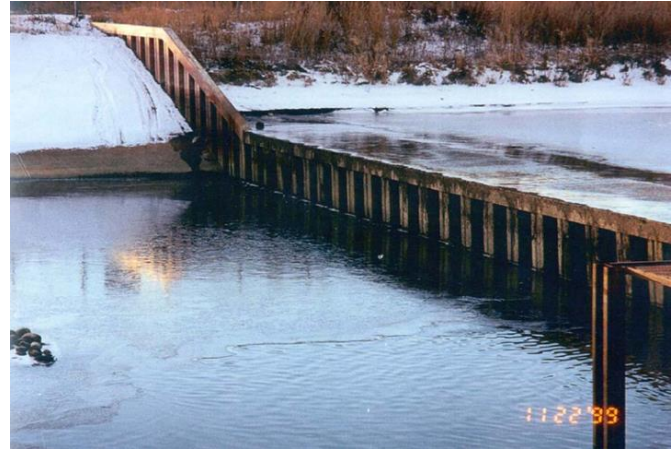
When the lake level drops below weir height, like in this 1999 picture, water ceases to flow in the Lesser Slave River, causing immediate negative impacts.
